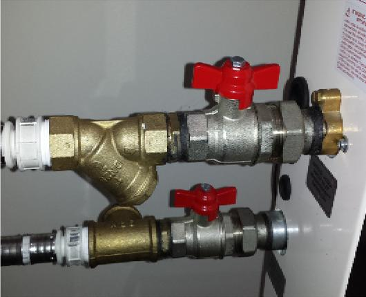
**Return:** Fit the union isolator and y-strainer to the upper 1" return connection on the appliance
