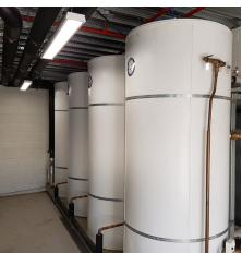
Sherwood Lodge Hot Water and Heating Skid: 80kW gas boiler and 1000 litres of storage.
