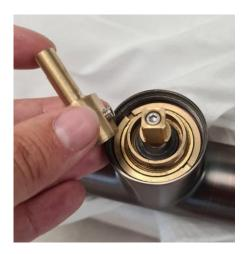
3. Remove brass locking nut that holds cartridge in place (it is threaded, but has flat edges to allow for removal by shifting spanner) – you should now be able to remove the cartridge.
