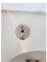
Note: when fitting the seat back onto the pan, make sure the seat is put back the same way it was removed, and that the spindles on the pan are lined up with the holes at the back of the seat.
