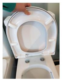
The spindles that the seats sit on will be visible – remove the chrome covers and locate the screws.
